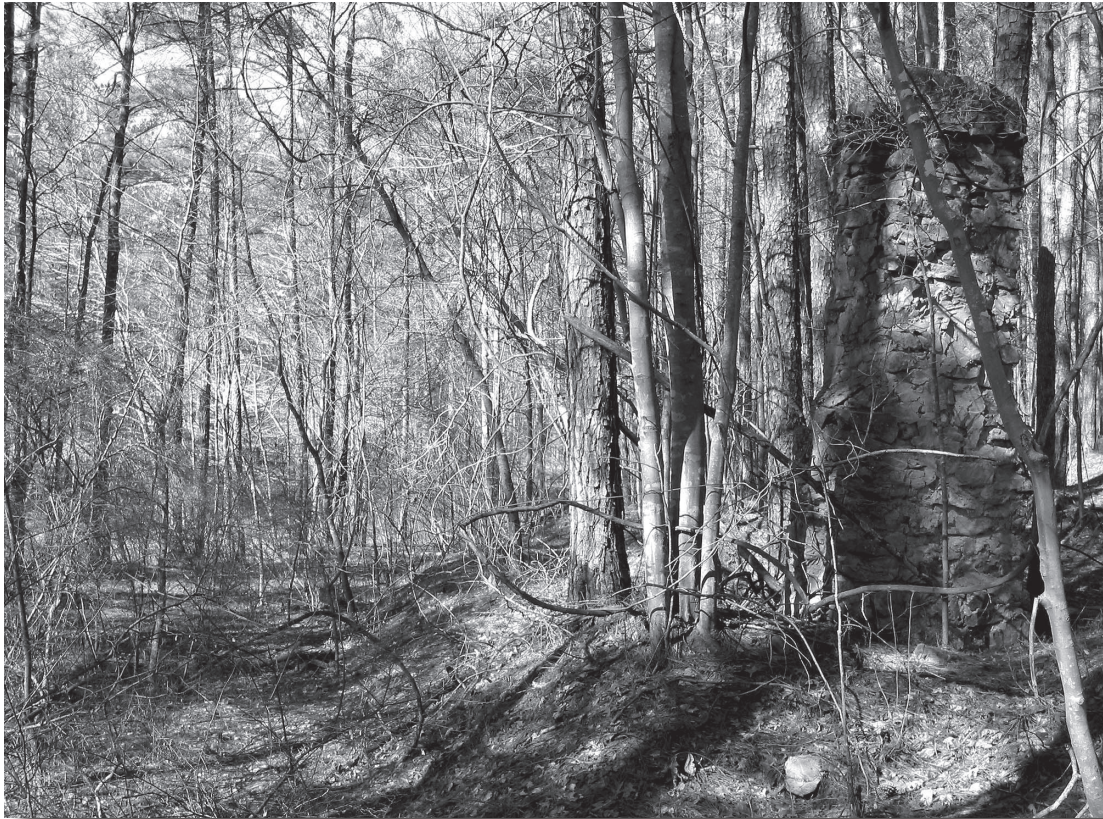
Old Smyer Lake Access Road and Relic Chimney
