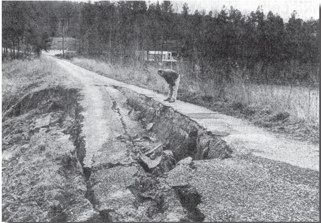
Hollybrook Dam Collapse, January 1990. Copyright © The Birmingham News , 2006. All rights reserved. Reprinted with permission.
